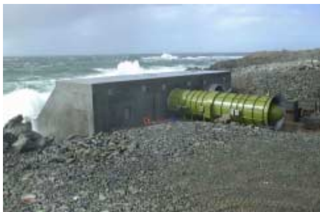
Figure 5.2 Landward view of 500 kW Scottish wave power technology at Limpet, Islay (source: Wavegen , 1999)
