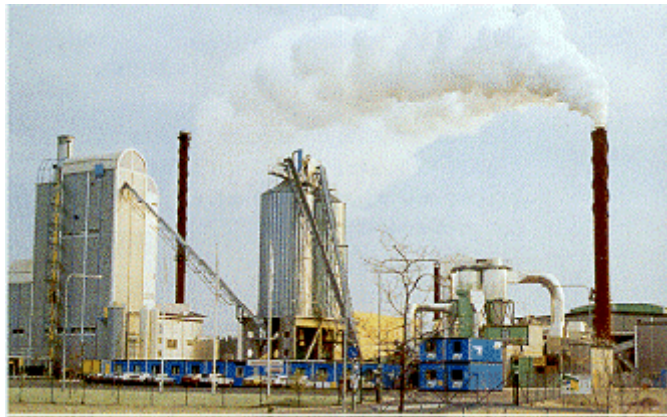
Figure 5.5 Biomass Electric power plant in Spain (source: http://www.europa.eu.int/ )
