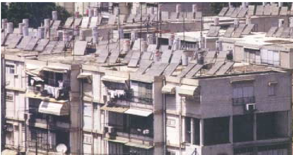
Figure 5.8 Domestic Water Heaters in Israel (Source: Renewable Energy World. Mar 2000)
