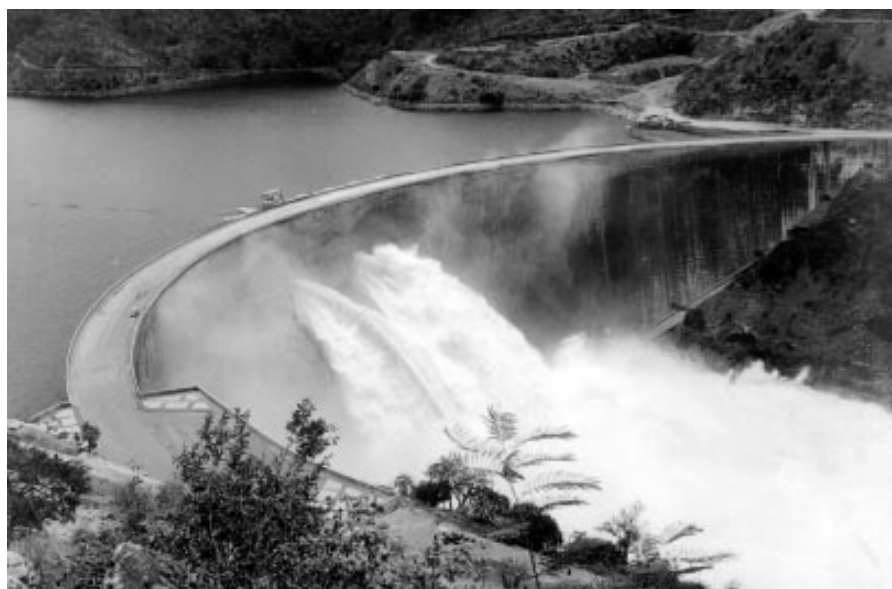
The Kariba Dam on the Zambezi, an example of regional collaboration in power generation between Zambia and Zimbabwe
